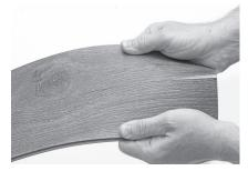
**Step 13** – Starting at one end, flex the vinyl plank up, then down - to snap it along the line.
